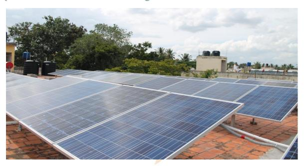
**Solar power plant** is based on the conversion of sunlight into electricity, either directly using photovoltaic(PV) and tracking systems to focus a large area of sunlight into a small beam. Photovoltaic converts light into electric current using the photoelectric effect.
